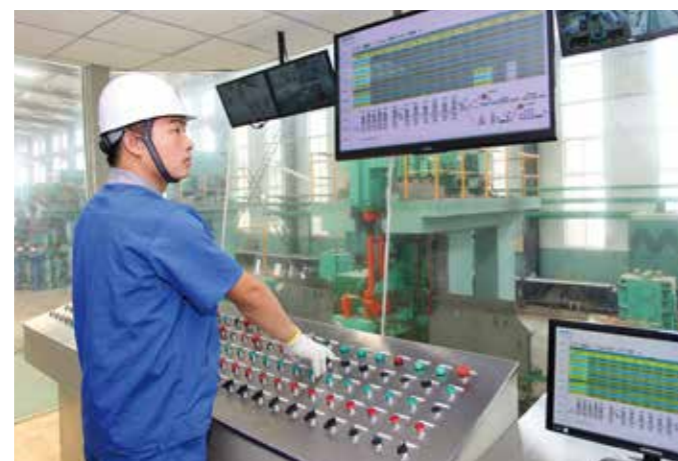
Continuous Rolling Mill Room
